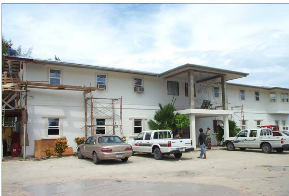
R&D/MIMRA building – photo taken on December 2001
