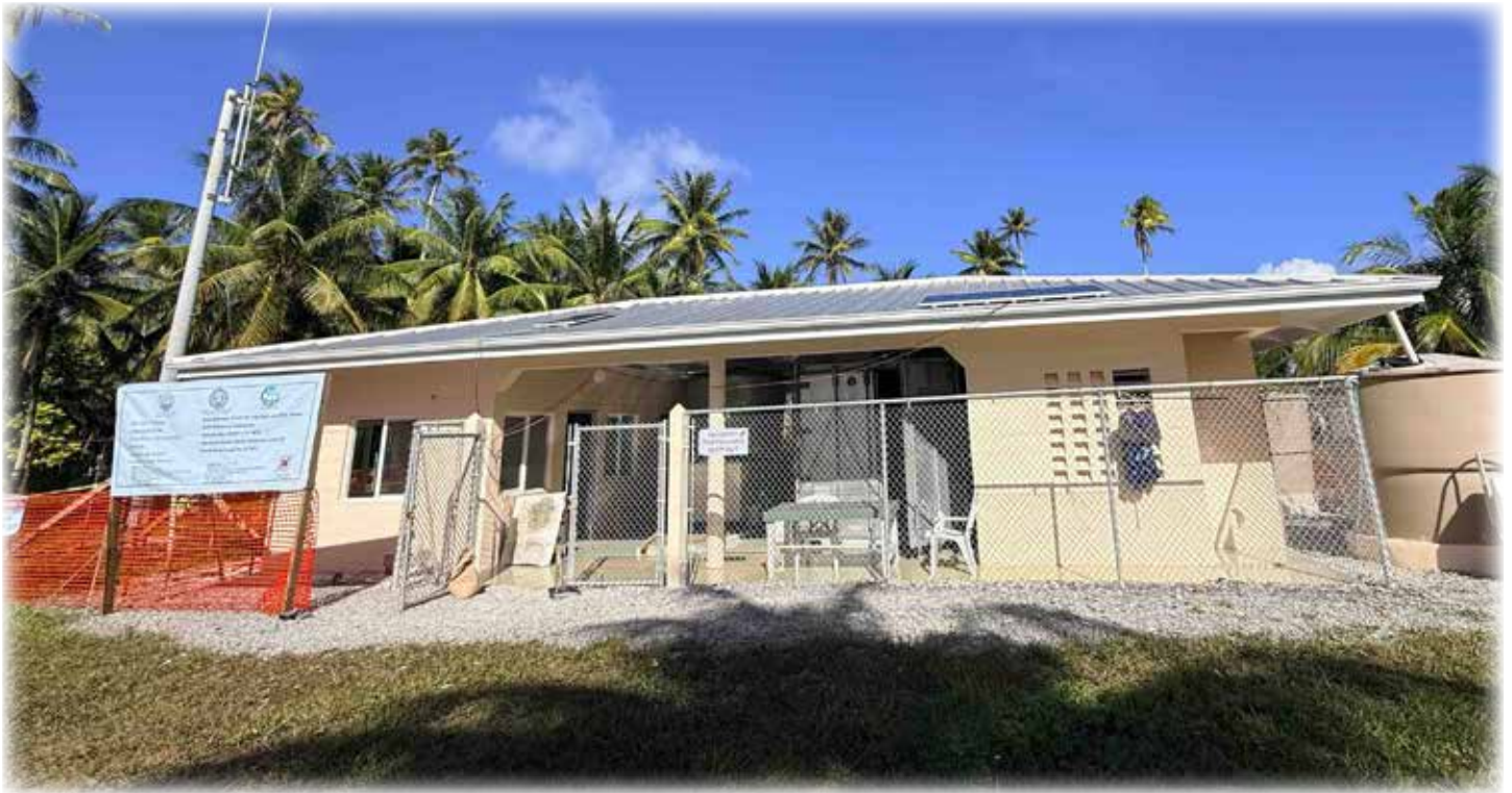
The Aur Atoll fish base received much-needed repair and maintenance.
