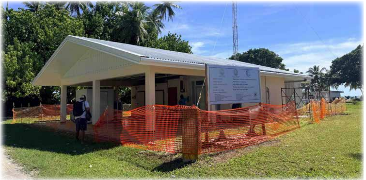
The Rehabilitation of fish bases is part of the World Bank's Pacific Islands Regional Oceanscape Program for Economic Resilience (PROPER). Pictured is the Arno fish base undergoing renovation.
